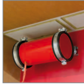
Fire extinguishing generator
