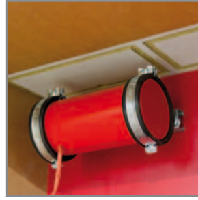
Fire extinguishing generator Current-independent tripping in the event of fire and impermissible temperature rise.
