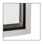
Housing ready for operation with smoke seal and safety glass
