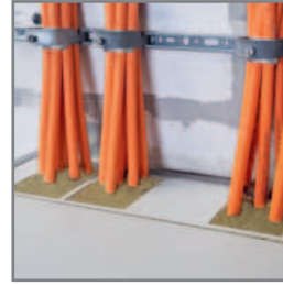
■ Cable insertion from above
