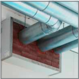
■ Pipe and cable bulkheads
