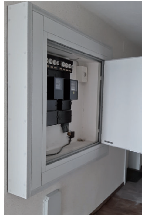
Retrofit fire-resistant panelling, in single or double-leaf design, over an existing, non-flush-mounted distribution system.
