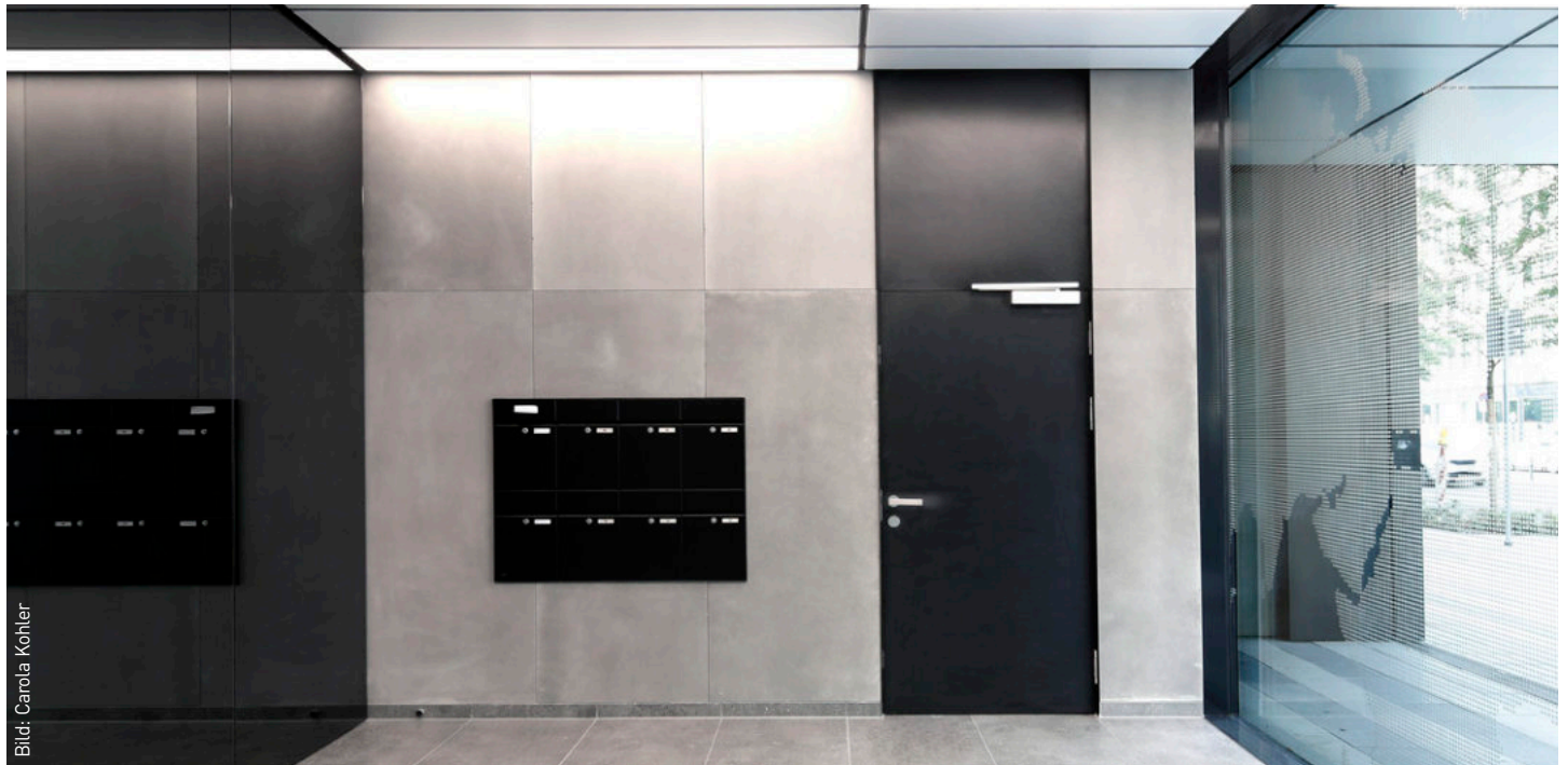
Fire protection closure clad on site for adaptation to an elegant ambience.
