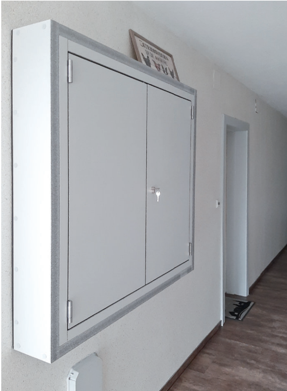
Retrofit fire-resistant panelling, in single or double-leaf design, over an existing, non-flush-mounted distribution system.
