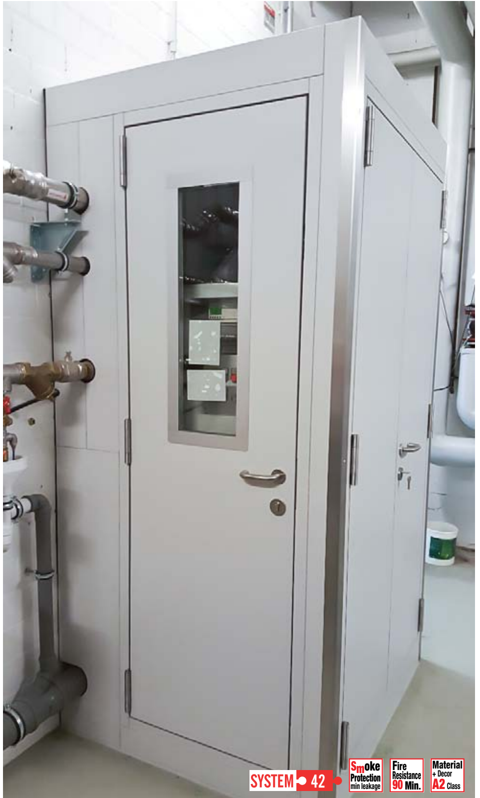
After the alterations
