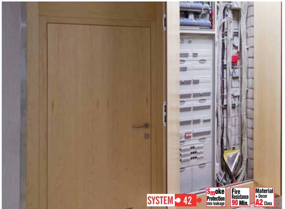
After the alterations
