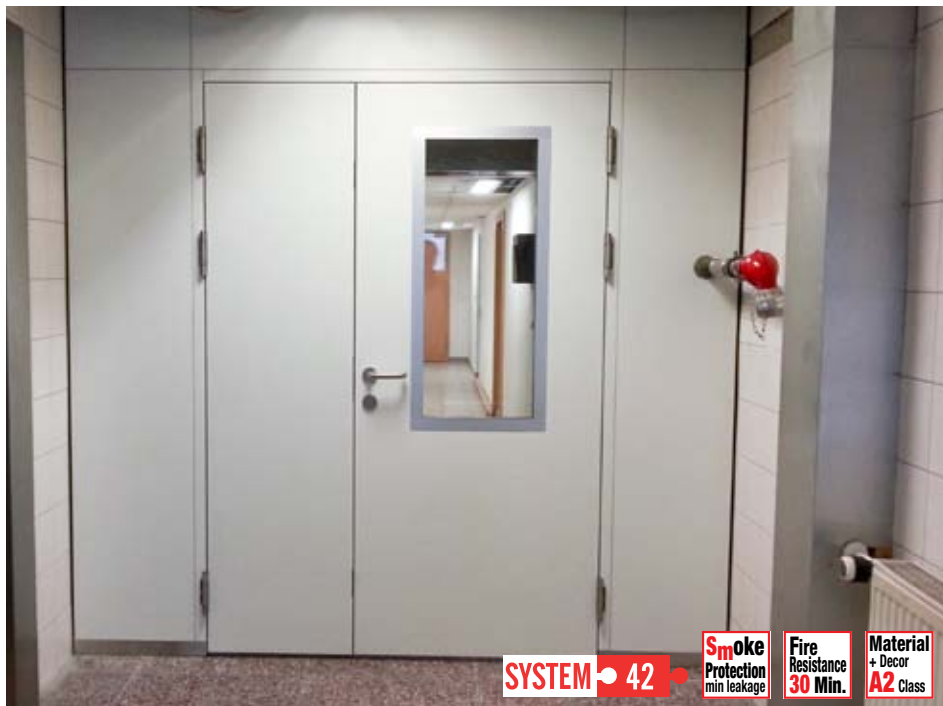
After the alterations
