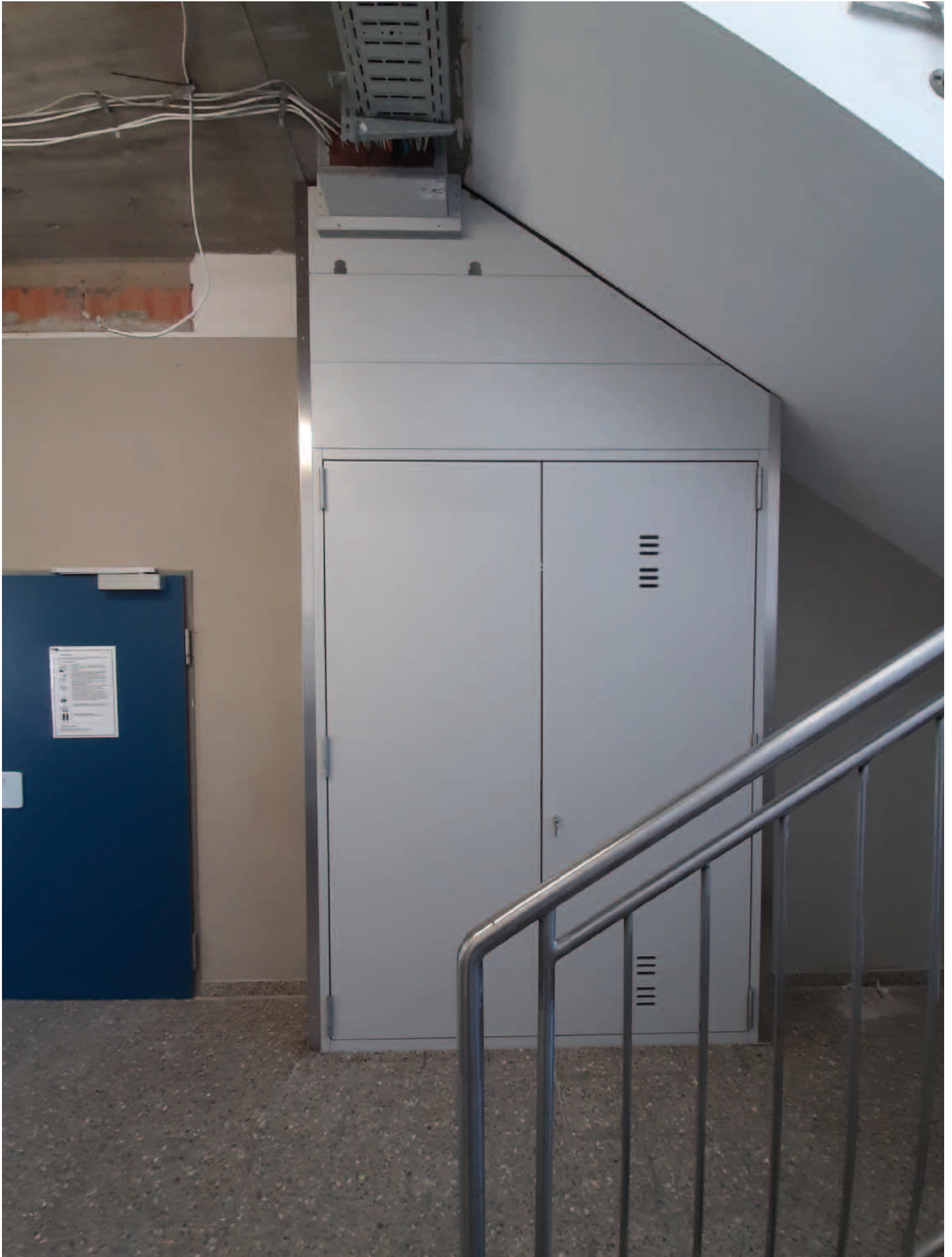
After modernisation: Fire-resistant wall system
