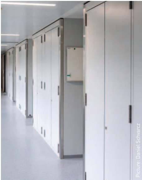
The prefabricated elements enable quick assembly
