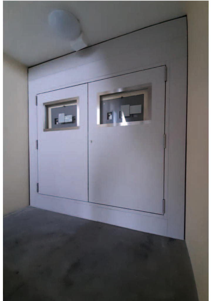
After modernisation: Fire-resistant wall system
