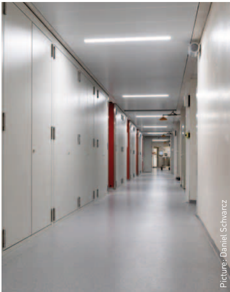
The individually planned and visually appealing wall systems with integrated inspection opening closures fulfil the fire protection requirements
