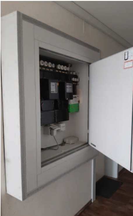
After modernisation: Fire-resistant wall system
