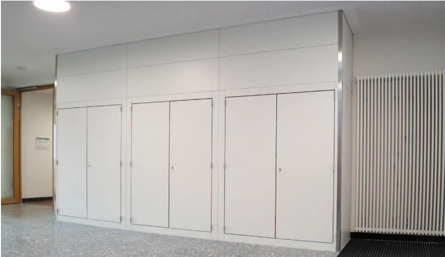
After modernisation: Fire-resistant wall system
