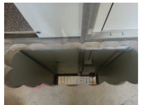
Core drillings for the construction of a smoke extraction shaft
