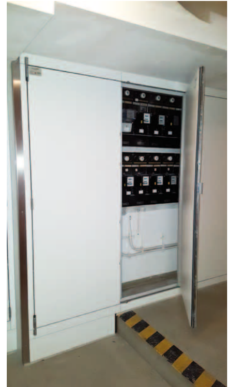
After modernisation: The fire-resistant wall system with large-format inspection closures offers safety and optimum accessibility to the electricity meters at the same time.
