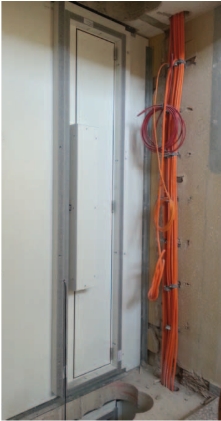
During the construction work: Construction of the smoke extraction shaft with wall elements only 42 mm thick
