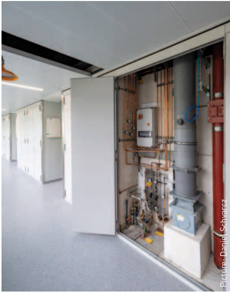
Electrical distribution boards, cables and ventilation and pipework were disconnected in accordance with current technical requirements, but remain accessible
