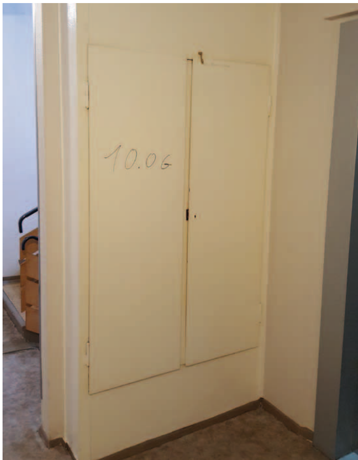
Before: Original panelling without fire protection classification
