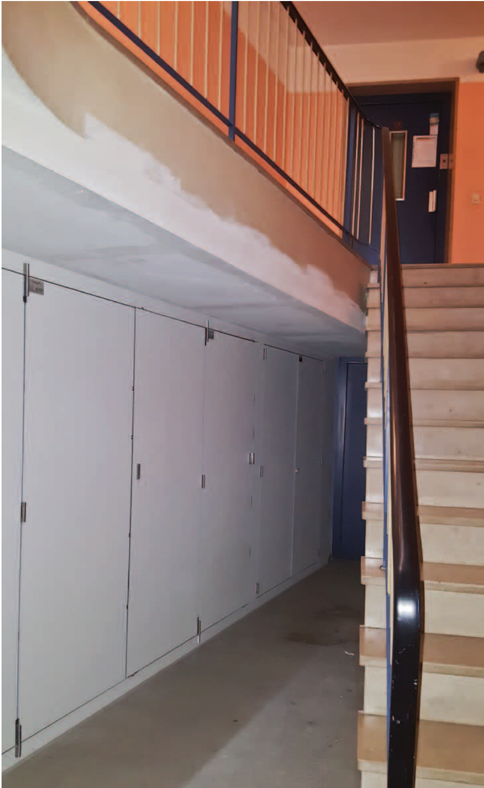
After modernisation: Fire-resistant wall system
