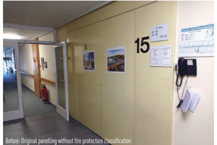
Before: Original panelling without fire protection classification
