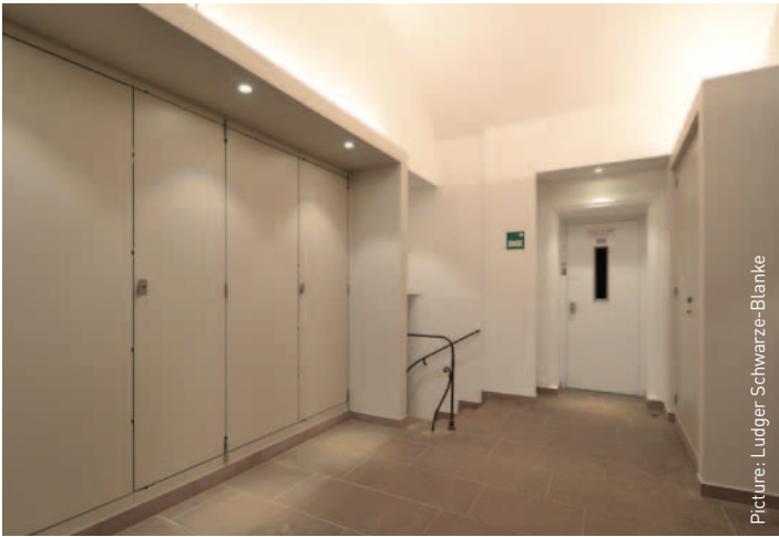
Cladding adapted to the colour concept protects the escape route from fire and smoke in the event of a fire in the electrical distribution system, while the large openings provide optimum accessibility.
