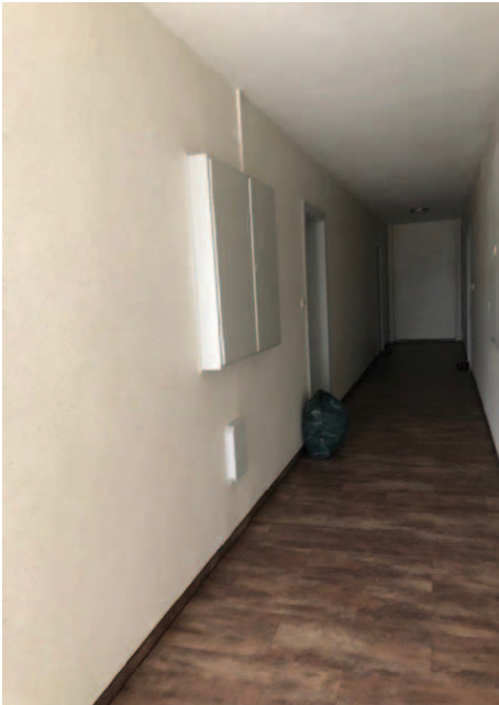
Before: Original panelling without fire protection classification
