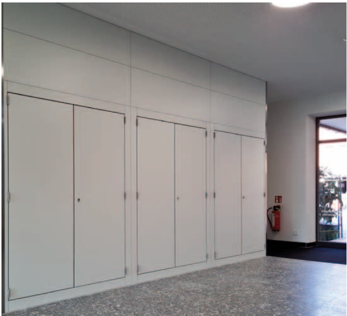
After modernisation: Fire-resistant wall system
