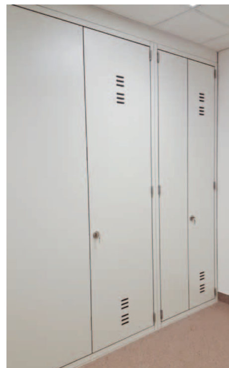
After modernisation: Fire-resistant wall system
