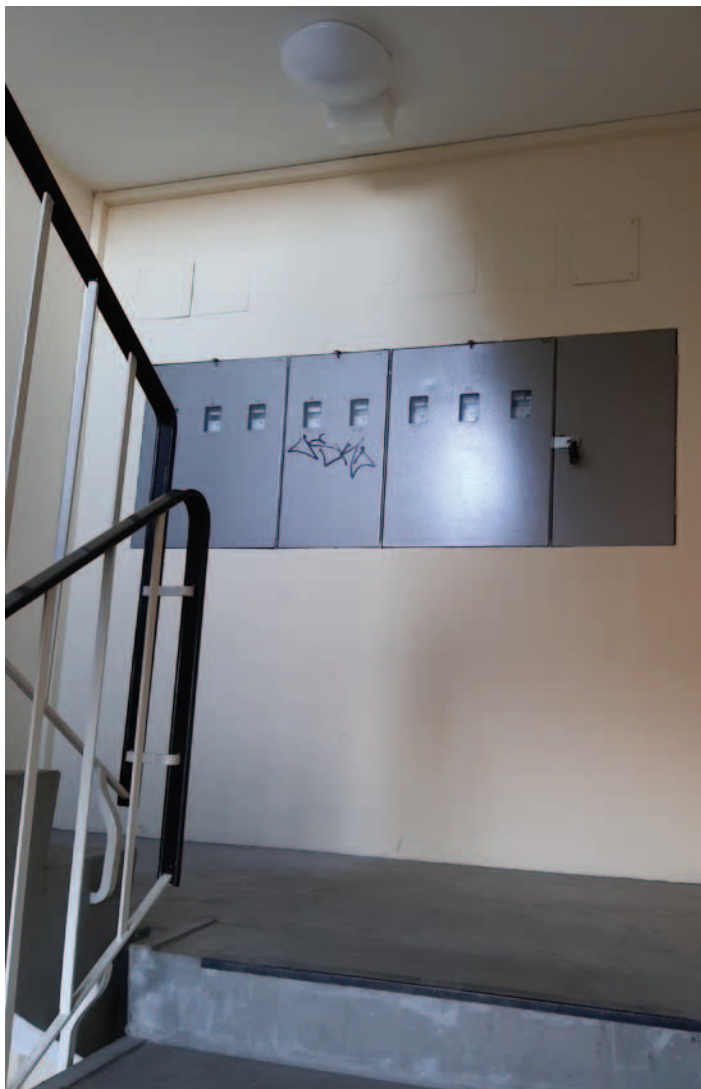
Before: Original panelling without fire protection classification
