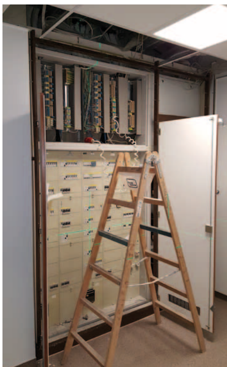
Before: Original panelling without fire protection classification
