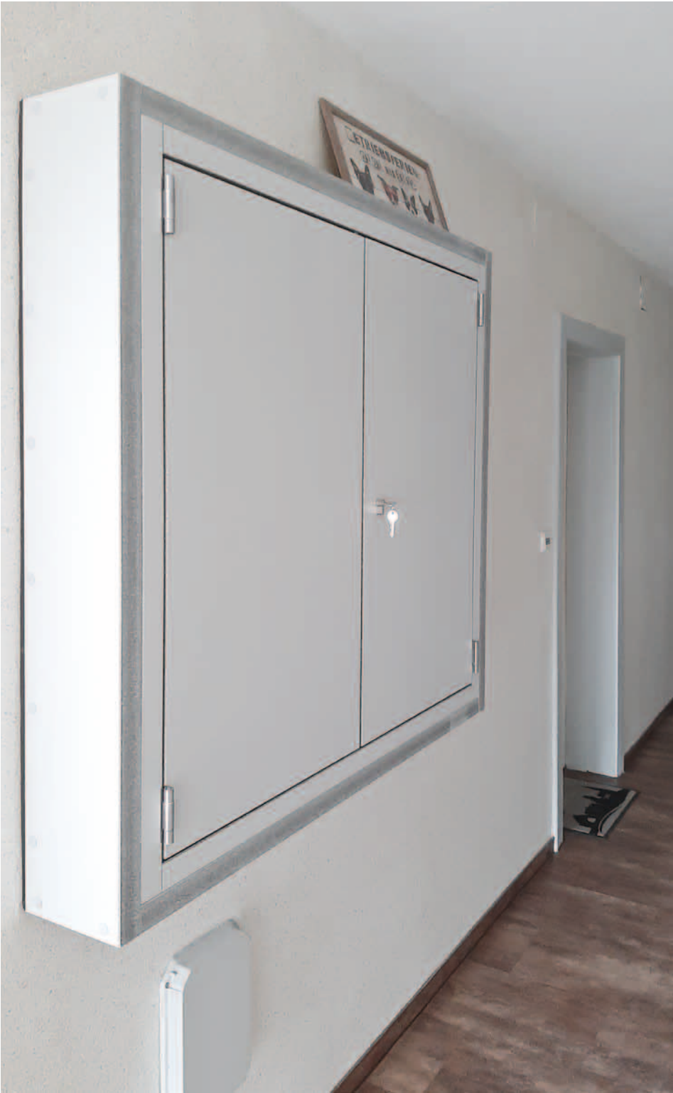
After modernisation: Enclosure with fire-resistant double-leaf inspection opening closures
