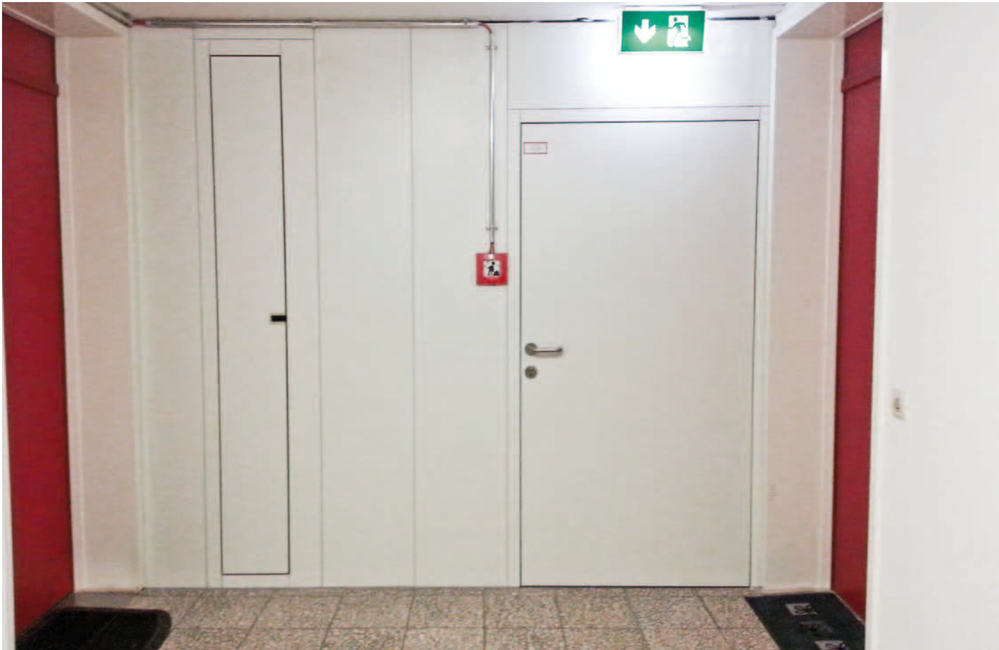
After modernisation: Fire-resistant wall system with smoke extraction flap and a fire protection closure (access door)
