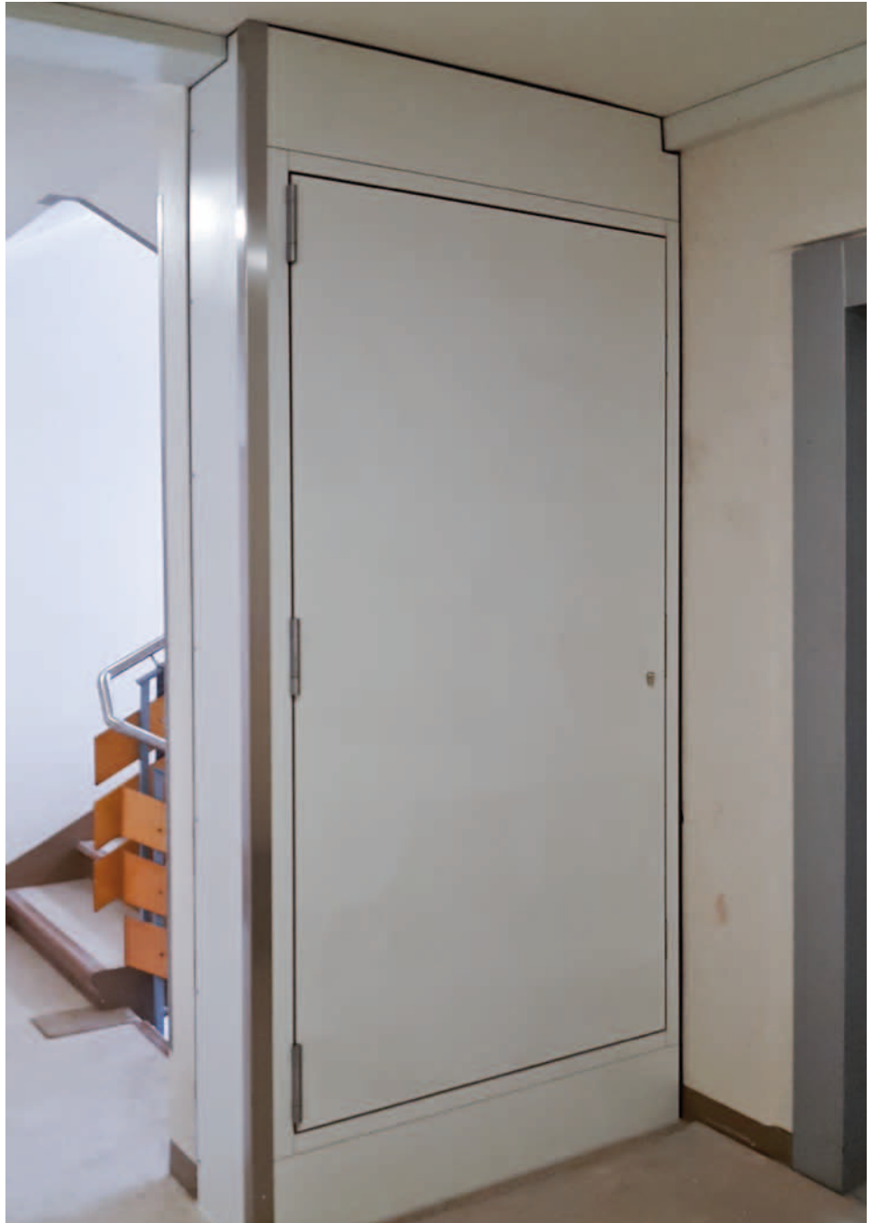
After modernisation: Fire-resistant wall system ensures optimum accessibility to the installations and at the same time offers protection against unauthorised access.
