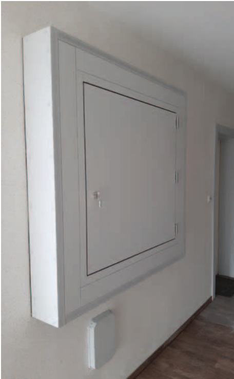
After modernisation: Fire-resistant wall system
