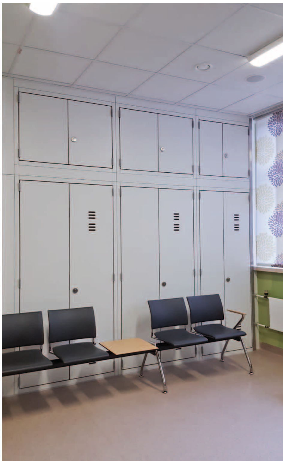
After modernisation: Fire-resistant wall system
