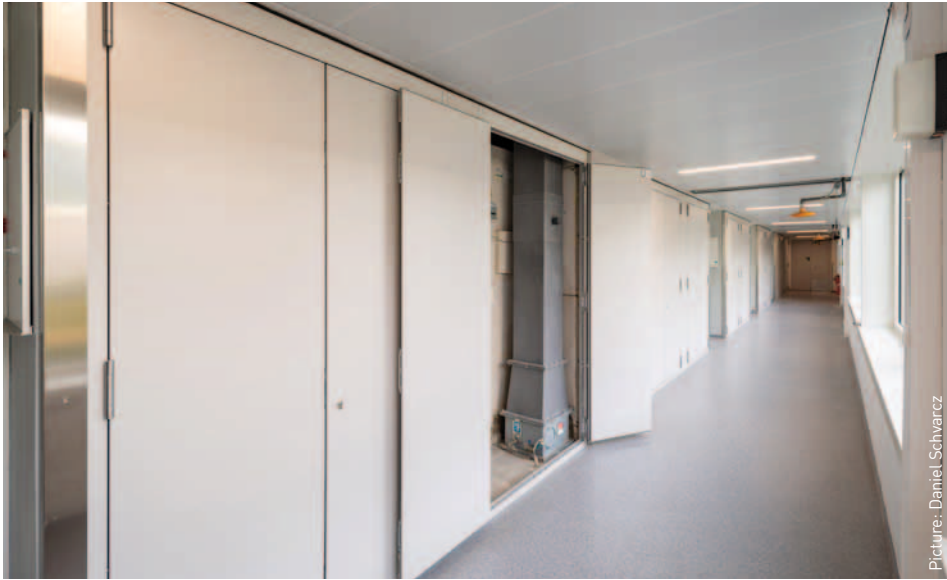
The wall system consists of single-layer, only 42 mm thick elements with a surface coating
