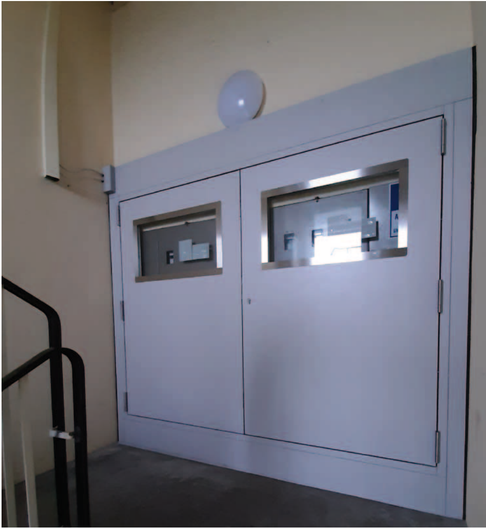
After modernisation: Fire-resistant wall system
