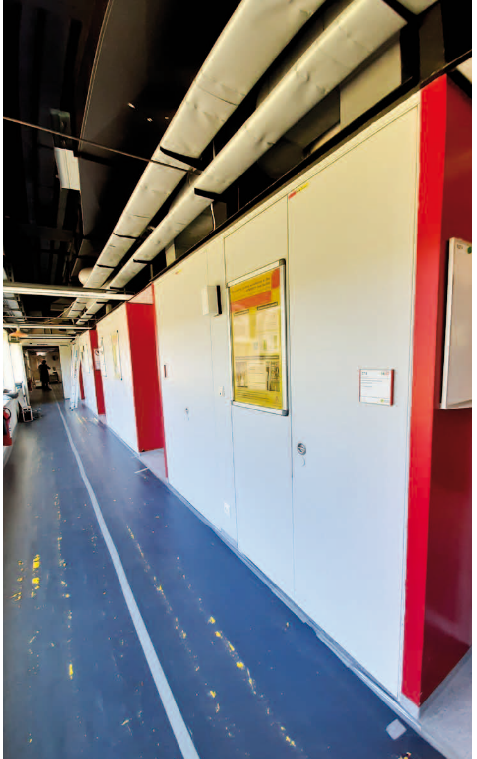
Before: Original panelling without fire protection classification
