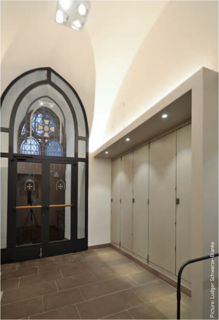
Finished panelling with inspection closures in a wide range of variants. From large-format to inconspicuous, visually adapted to the respective requirements, they enable almost optimal accessibility for subsequent occupancy or maintenance work
