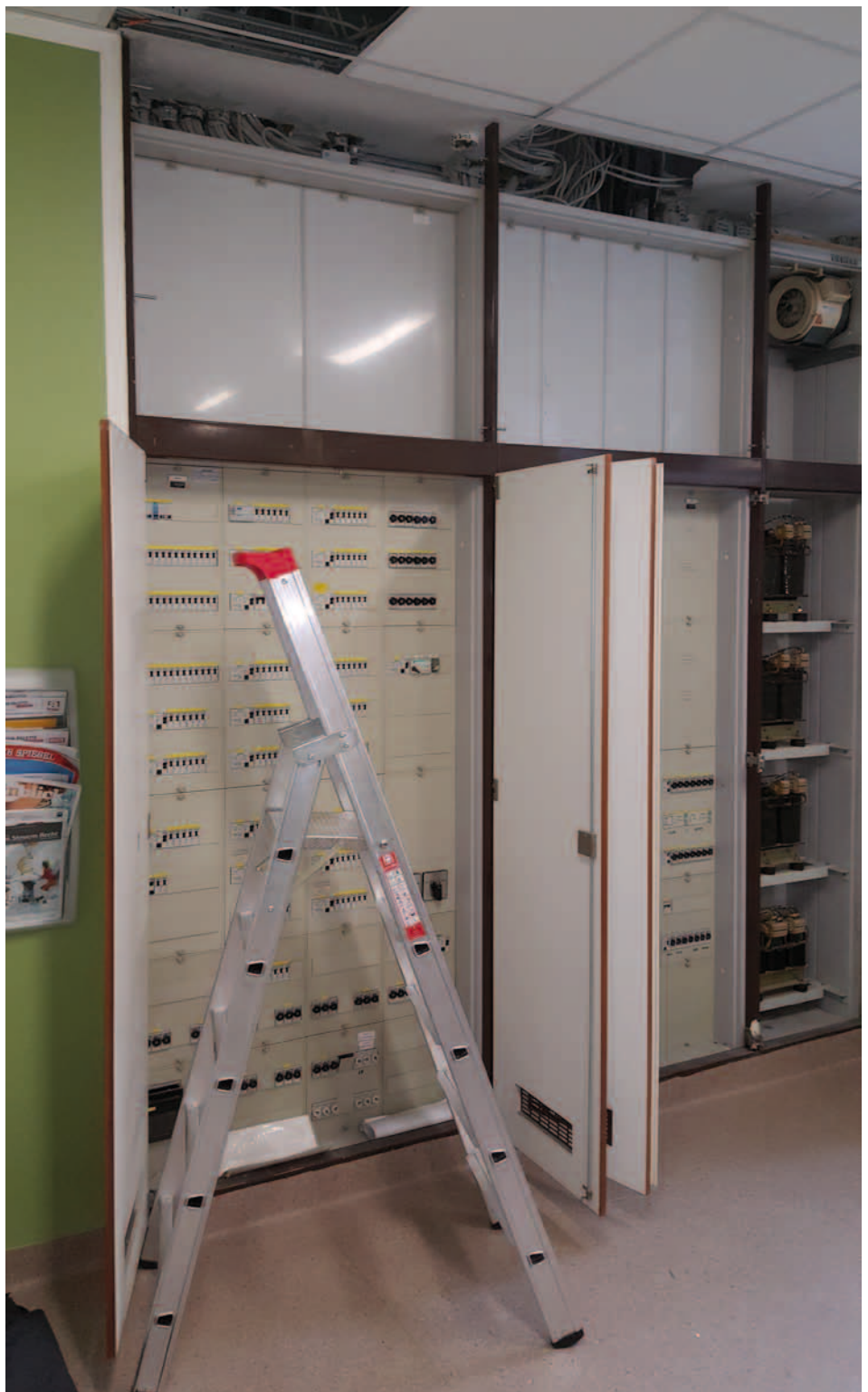
Before: Original panelling without fire protection classification
