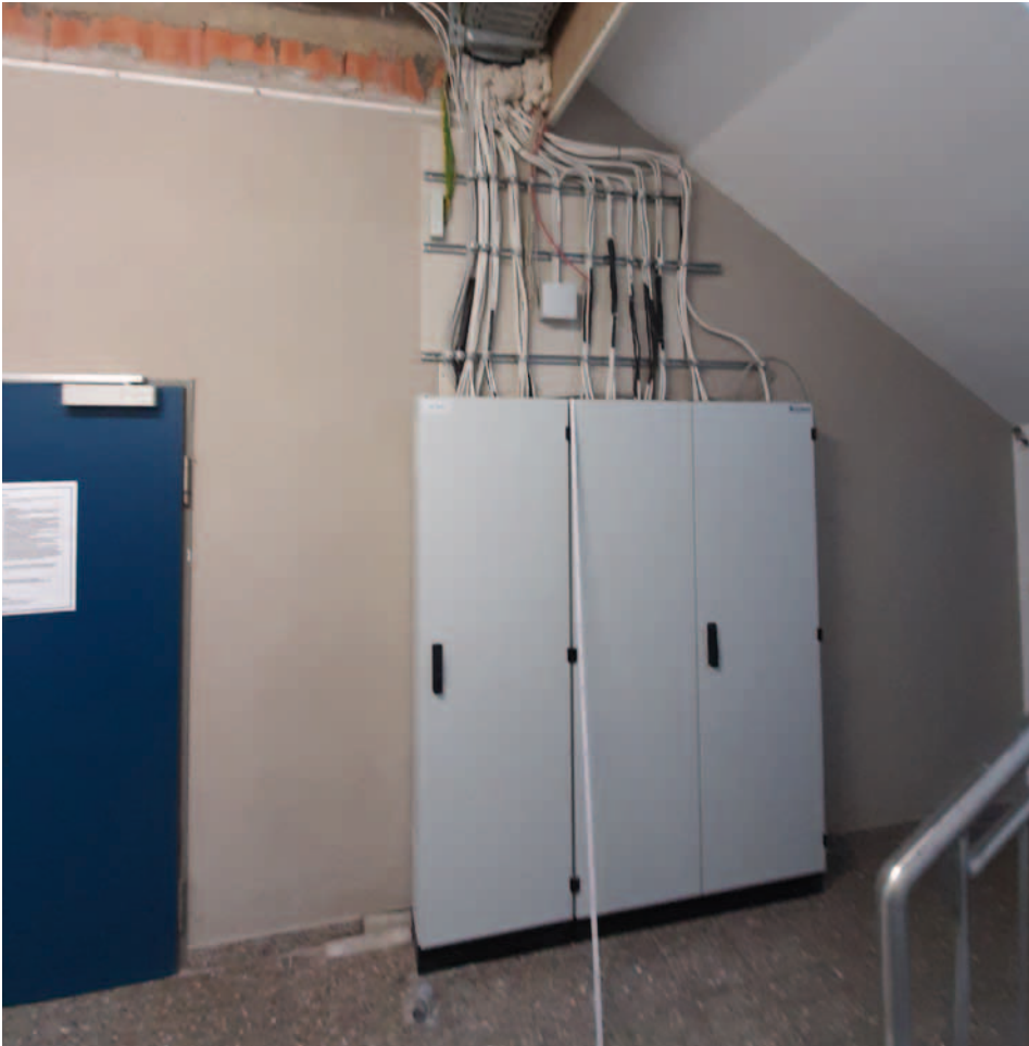
Before: Original panelling without fire protection classification
