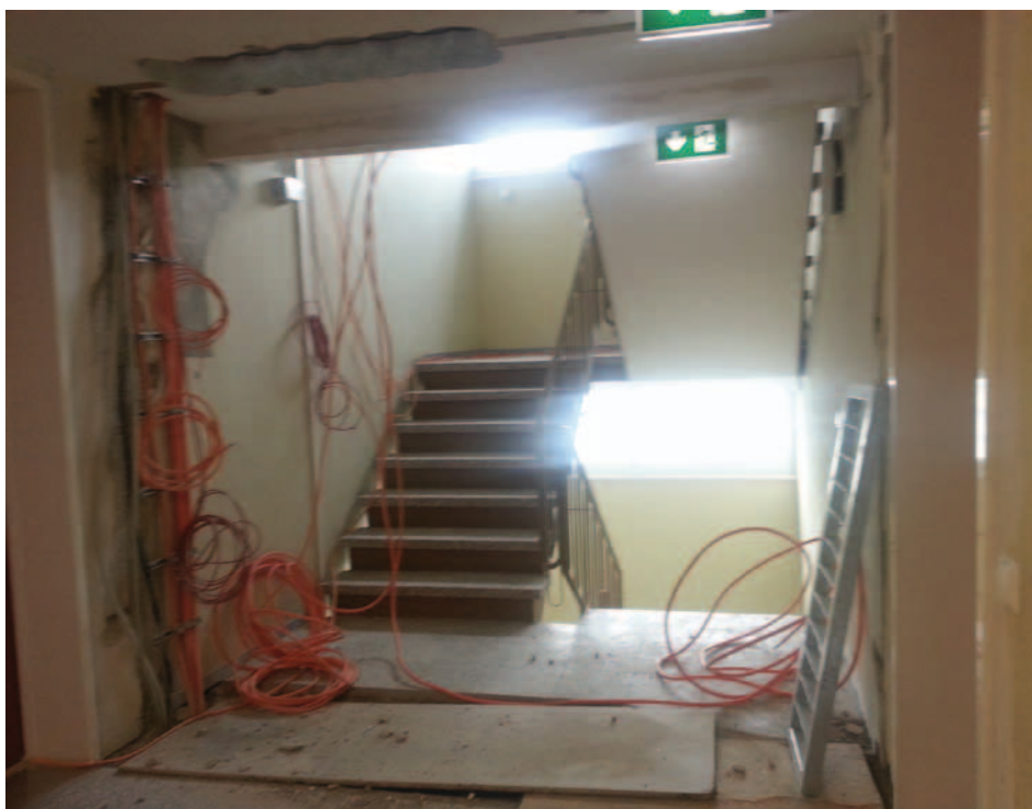
During the construction work: Dismantling of the existing panelling
