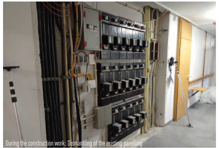
Before: Original panelling without fire protection classification
