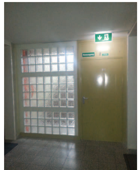
Before: Original panelling without fire protection classification
