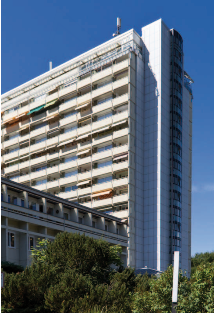
Before: Original panelling without fire protection classification
