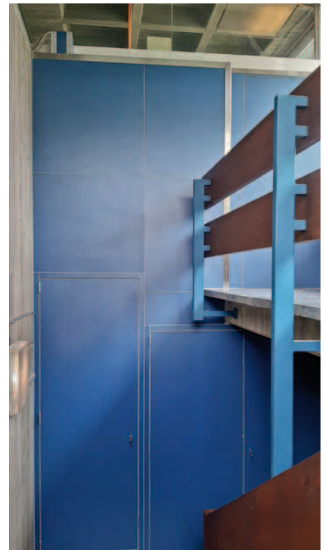
Precisely prefabricated elements, special colour similar to RAL 5000; wall elements can be individually adapted to the structural conditions on site.
