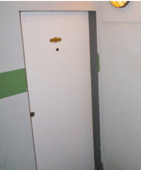
Before: Original panelling without fire protection classification
