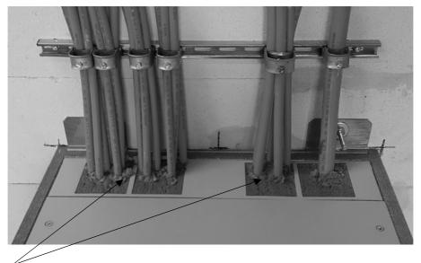
After cable installation, the existing gaps must be stuffed with mineral wool to achieve protection class IP 44.
