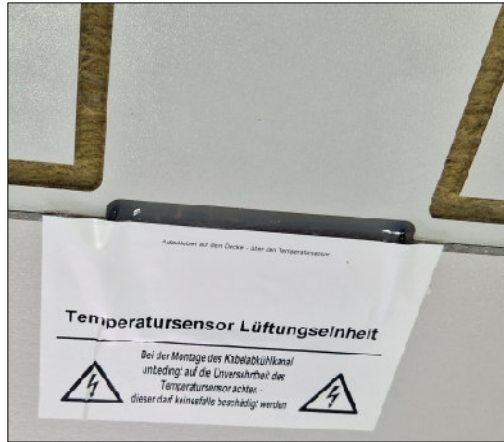
Figure 20, Sealing temperature sensor cover element
