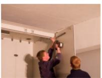
• Install the door closer and slide rails based on the manufacturer's instructions. Holes are pre-drilled for this purpose.
