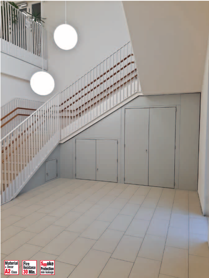
Fire-resistant partition, L-shaped design, the prefabricated elements enable quick assembly
