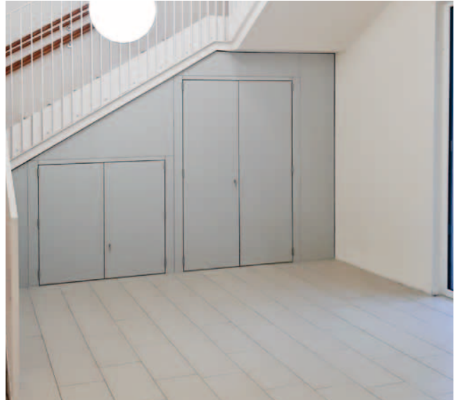
After the refurbishment - PRIOWALL wall system with large-format access panels
