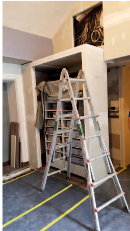
Fire-resistant enclosure of fire loads - drywall construction in combination with elements of System 42 by PRIORIT
