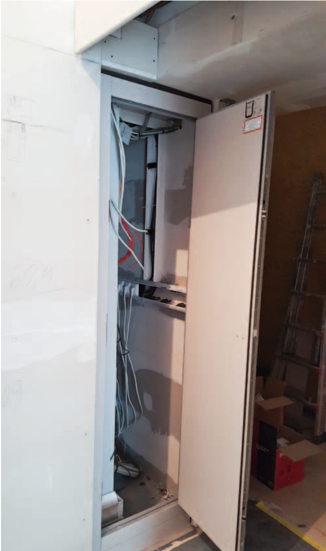
Inspection closure with all-round frame in the same look ensures accessibility
