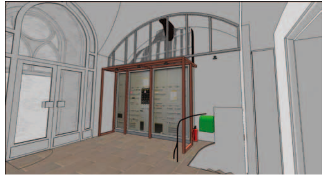
Steel scaffolding to form the drywall construction
