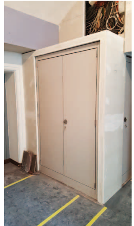
Fire-resistant enclosure of fire loads - drywall construction in combination with elements of System 42 by PRIORIT
