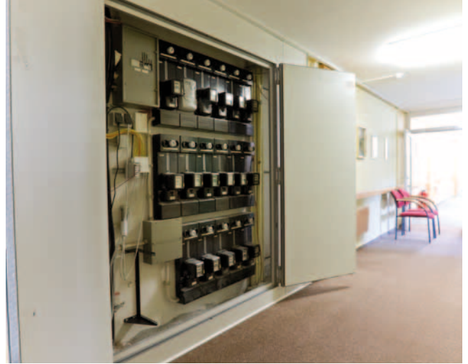
After the conversion work
