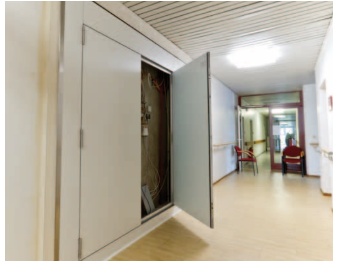
After the conversion work
