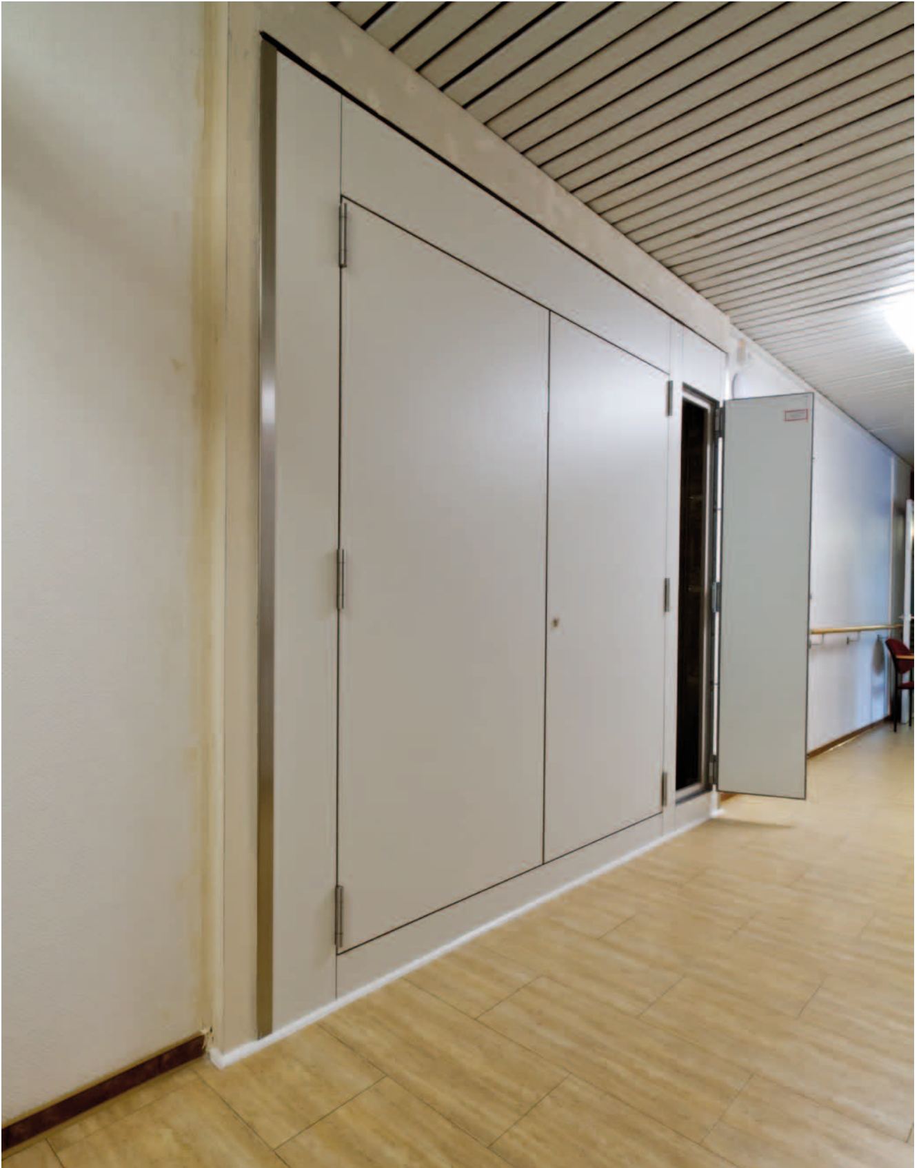
After the conversion work
