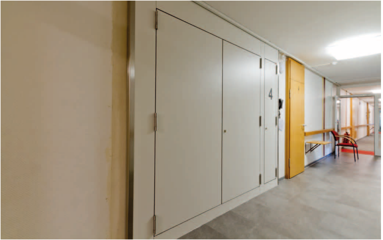
After the conversion work
