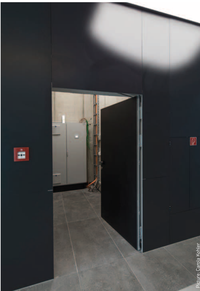
Fire protection closure installed in a solid wall, with cladding applied on one side by the customer
