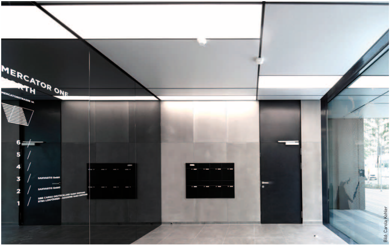
Fire protection closure clad in uniform metal finish
