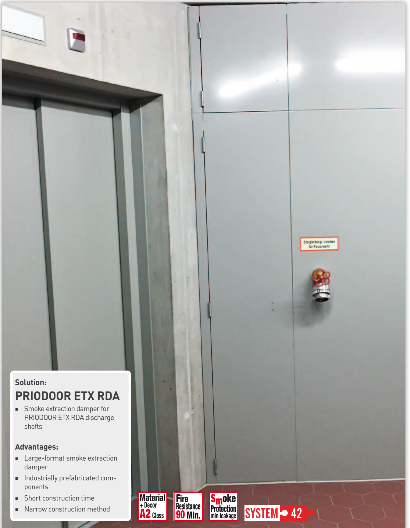
PRIODOOR ETX RDA smoke extraction damper
