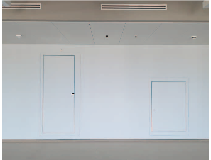
PRIODOOR ETX RDA smoke extraction damper and PRIODOOR RTH inspection opening closure arranged next to each other. Discreet and unobtrusive while complying with all functional and safety requirements
