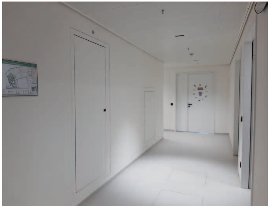
Large-format smoke extraction damper and inspection cover with a standardised appearance, adapted to the structural specifications of the overall concept
