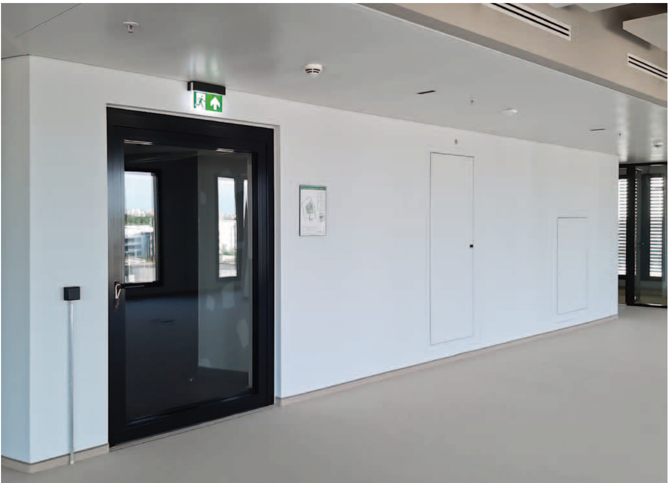
PRIODOOR ETX RDA smoke extraction damper and PRIODOOR RTH inspection opening closure arranged next to each other. Discreet and unobtrusive while complying with all functional and safety requirements
