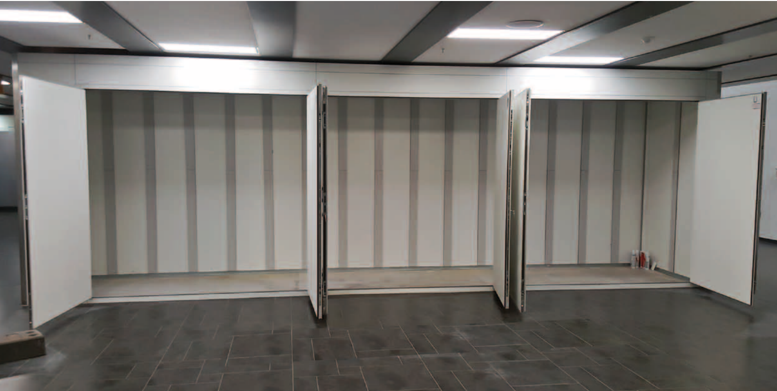
The door-to-door design with a low centre bar allows almost complete access to the room for installation or maintenance work
