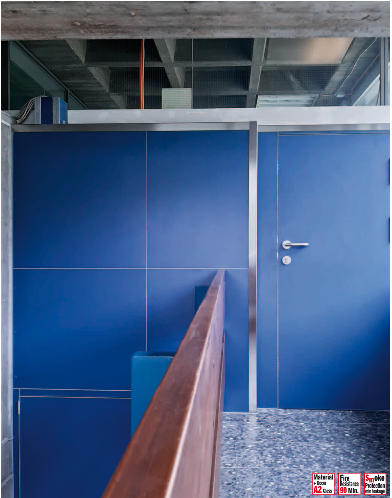
PRIOWALL wall system with PRIODOOR ETX inspection opening closures and PRIODOOR FSA fire protection closure in Alpine blue for separating electrical distribution boards and fire compartments in the escape route.
