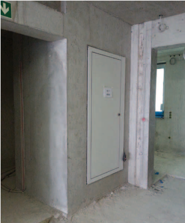
Installation of the smoke extraction damper during the construction phase
