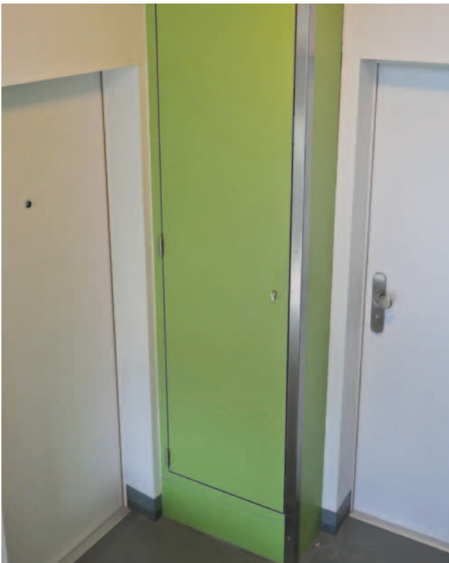
After modernisation: PRIOWALL with a fire resistance rating of over 90 min. - Version in decorative surface green similar to RAL 6024
