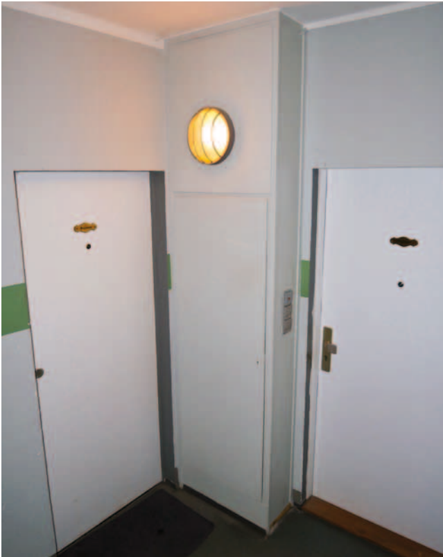
Before: Original panelling without fire protection classification
