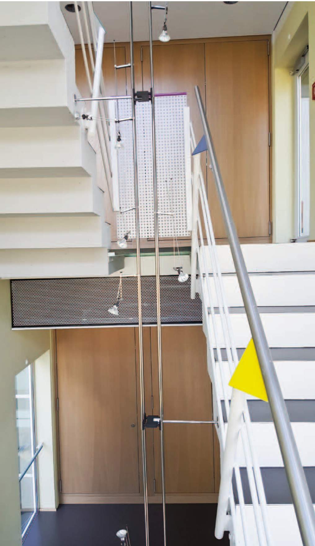
Fire-resistant, non-combustible wall construction system with integrated inspection opening closures in the stairwell
