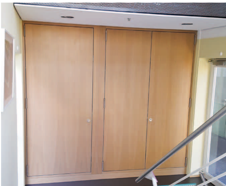
Fire-resistant, non-combustible wall construction system with integrated inspection opening closures in the stairwell
